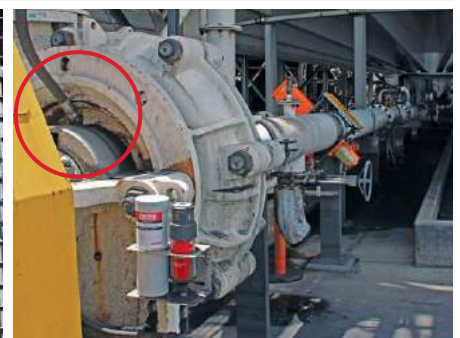
Pump bearing lubrication
