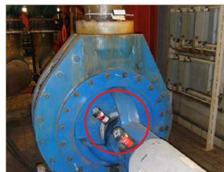
Lubrication of drive shaft on pump
